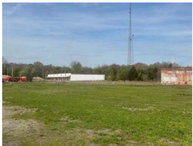
221-051-07 – FORMER MILL BUILDINGS
