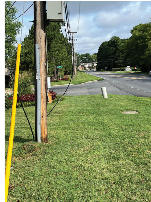
Utilities along the path of the new sidewalk. View is looking north across Sable Park Drive.
